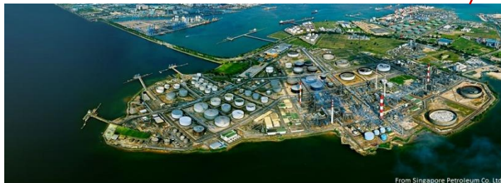
Industrial and Petroleum Industries
